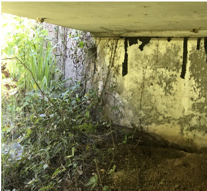
PHOTO 1 Description Bent 1 Rt spalling with exposed reinforcing steel in the end of the abutment.
