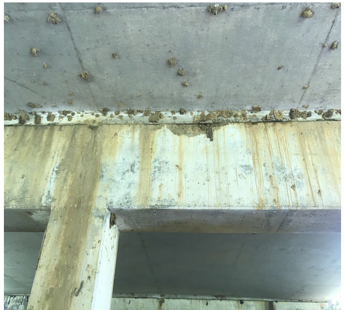
PHOTO 2 Description Bent 2 Span 2 shallow spalling in the bearing area.
