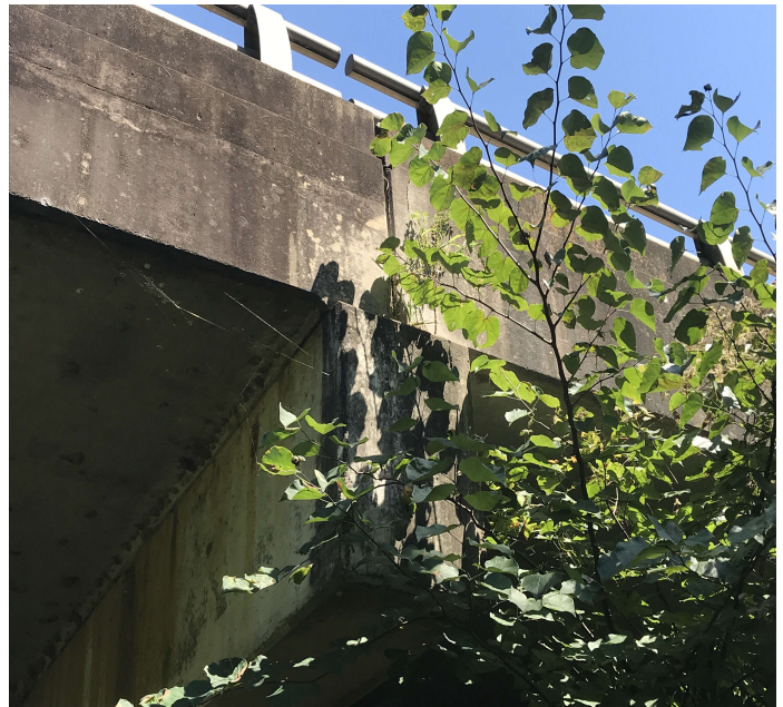
PHOTO 2 Description Span 1 @ Bent 2 Lt Vertical crack in the edge of the slab.
