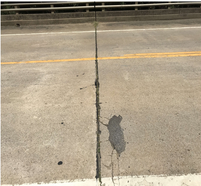
PHOTO 1 Description Bent 2 failing joint seal.
