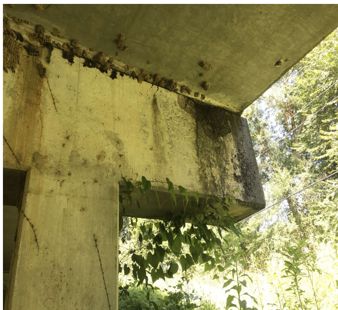
PHOTO 3 Description Bent 3 Rt spalling with exposed reinforcing steel.
