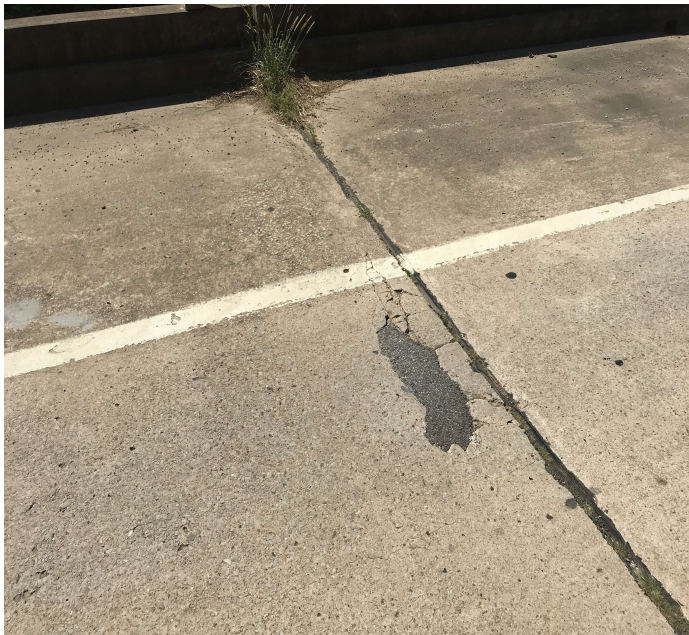
PHOTO 1 Description Span 1 Lt spalling and delaminated concrete adjacent to the deck joint.
