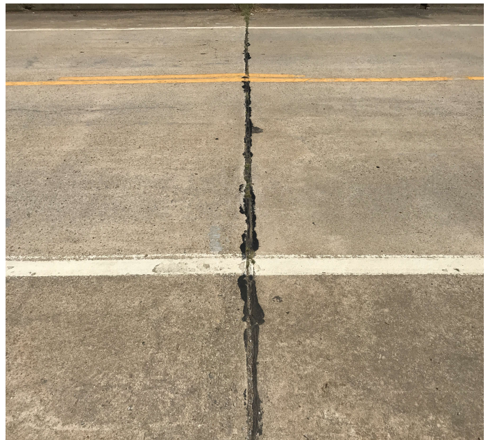
PHOTO 2 Description Bent 3 failing joint seal.
